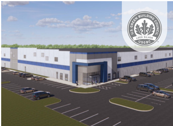
CROSSROADS 95 LOGISTICS CENTER, NEWARK, DE 442,530 SF
