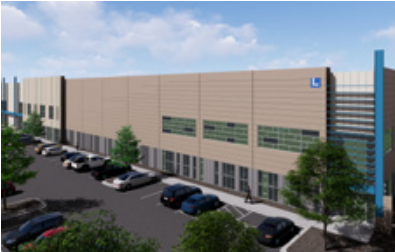
EAGLE 25 LOGISTICS CENTER, THORNTON, CO
