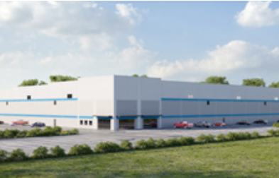
UNITED LOGISTICS CENTER, WEST BRIDGEWATER, MA
