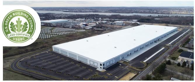
BOX PARK LOGISTICS CENTER Cinnaminson, NJ | 1.2M SF
